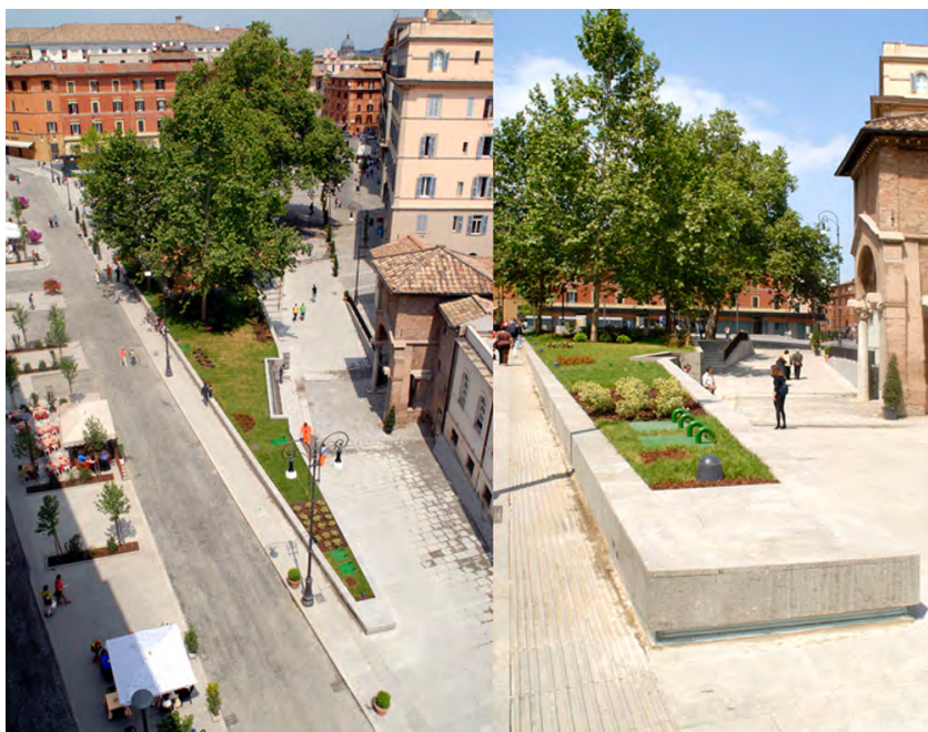
Fig. 1. Prothyrum, hospital entrance and square after redevelopment, 2009 20 .
